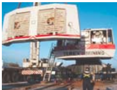
Assembly of the counterweight
