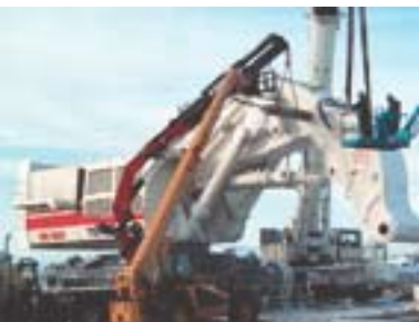
Connection of boom and stick
