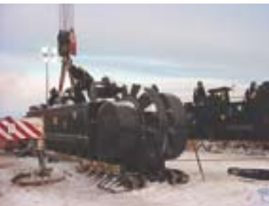
Positioning of the crawler frames
